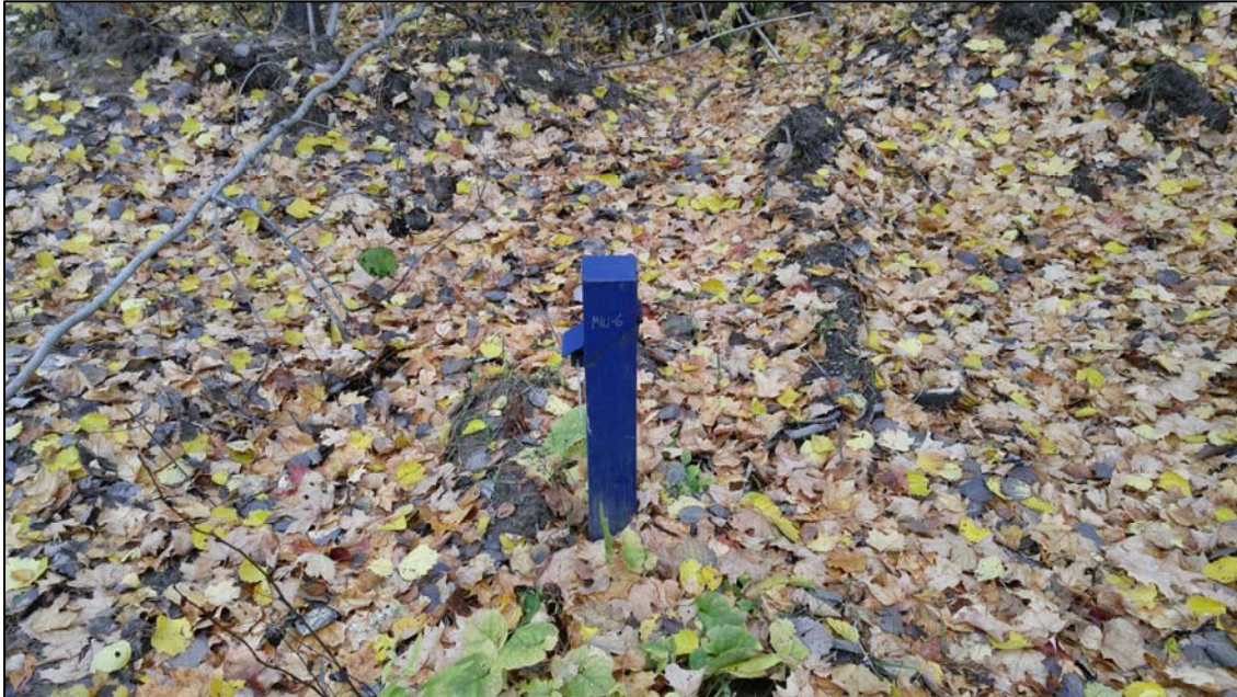
PHOTO 5 – MW6 Monitoring Well (Fall 2020).
