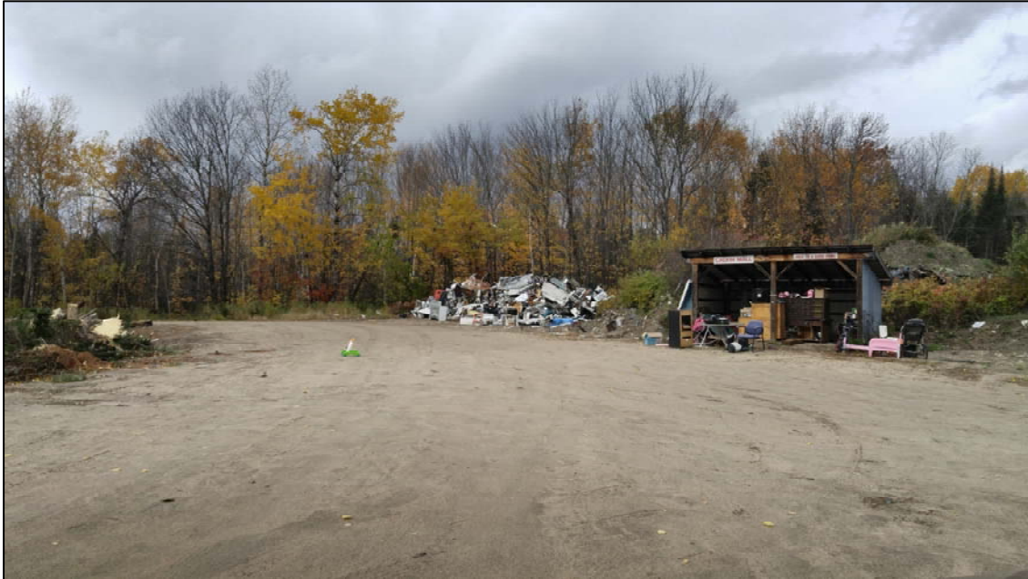
PHOTO 13 – General Site Picture (Scrap Steel and Calvin Mall) (Fall 2020) .
